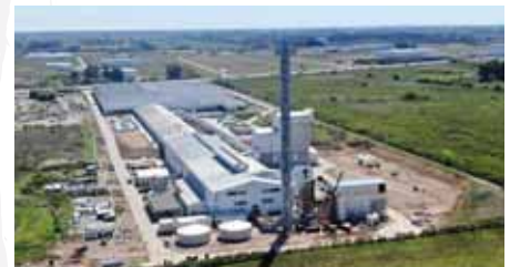
The new plant at Los Cardales, Argentina
